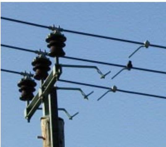
**Picture 3.** Suspension pole with oscillating clamps and lightning protection.
