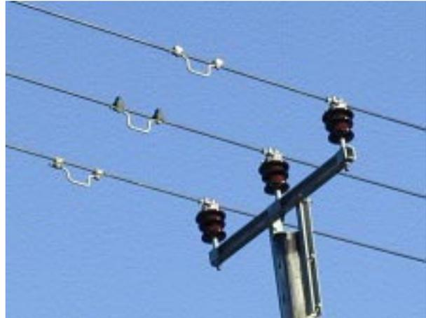
**Picture 4.** suspension pole with earthing stirrups.
