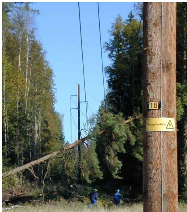
Figure 7. Falling tree test in Forest-Sax line.
