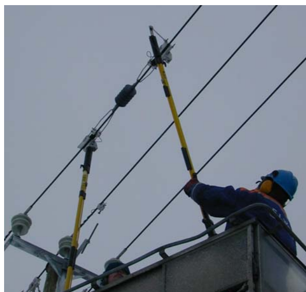
Figure 4. Live line disconnection point under work.
